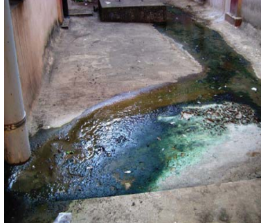
Sewage surrounding new hospital
