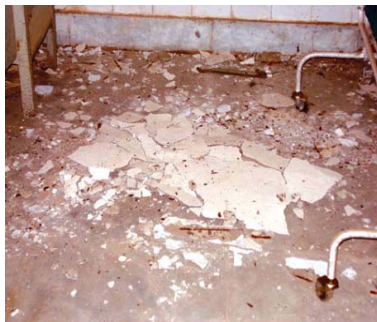
Ceiling cement in new operating theater floor
